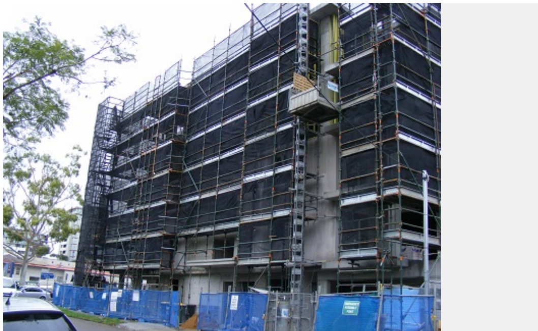
Construction on Conder Street, Burwood.
